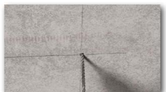
1 Drilled hole Ø 6 mm.
