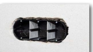
**4** Insert box in wall and protect with signal covers (p. 45).
