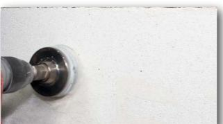
**2** Cut holes with milling bit.
