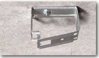
**5** After fastening, the multi bracket can be directly equipped with cables and wires.
