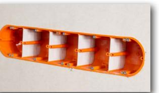
**3** Insert box and secure it with screws.
