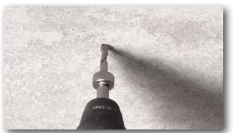
**1** Pre-drill a defined hole with a stop drill.
