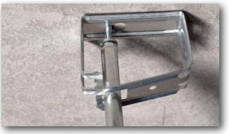
**4** Drive in the dowel in one step using the hammer function and thus fasten the multi bracket.
