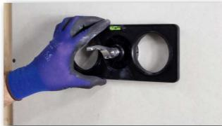
2 Precise alignment with the integrated spirit level and fastening of the drilling template with the tensioner.
