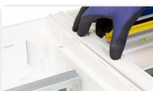
6 Insert the connected distributors as one unit into the wall, tighten the hollow wall anchor and click the end rail onto the gap from the front.
