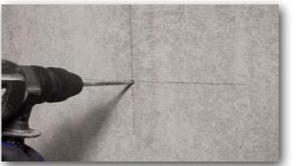
1 Drilled hole Ø 6 mm.
