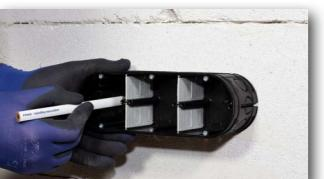
**1** By marking the holes, centering points are marked out.
