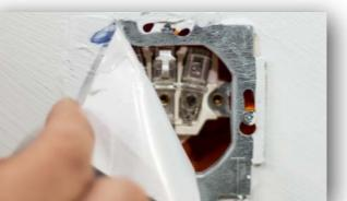
**6** After the work, remove the f-Sticker without leaving any residue.
