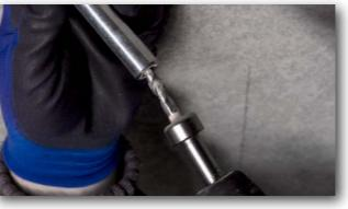
**3** Place the setting tool on the drill and set to hammer.
