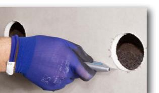
**2** With mill bit Ø 68mm cut, make the two outer holes and cut out the centre piece using a cutter or jigsaw.
