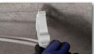
2 Simple installation of the anchor system (CMS 5, 6, 7 or 8). Insert the collection holder.
